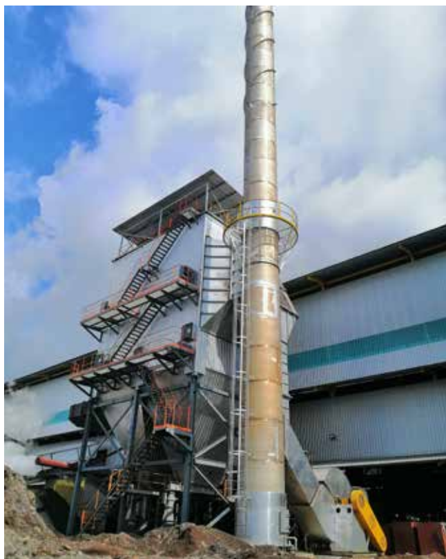
Electrostatic precipitator (ESP) for Boiler Flue Gas Filtration at TBS Oil Mill
